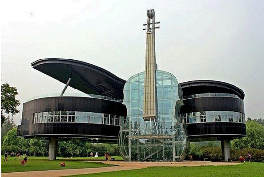
piano house . Huainan, China.
